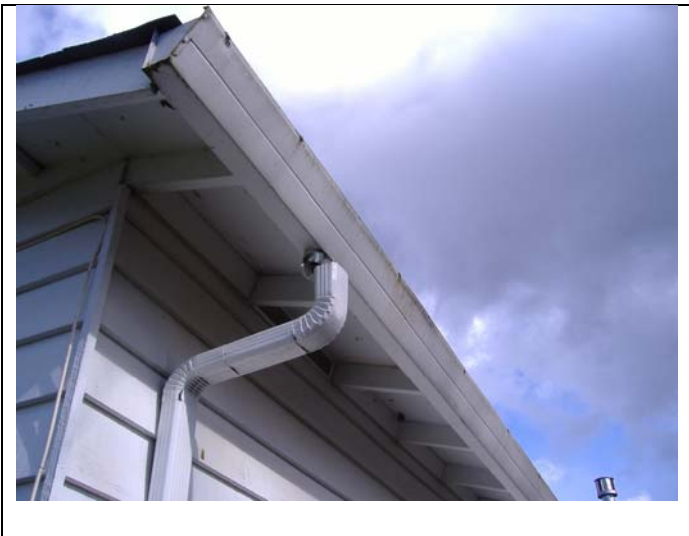
Downspout disconnected.
